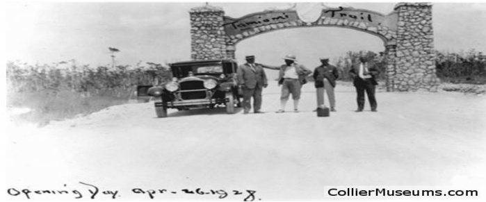
Archway between Collier & Dade County on the opening day of the Tamiami Trail.
