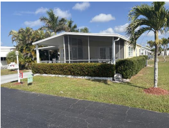
Manufactured home with gutter that drains away from property
