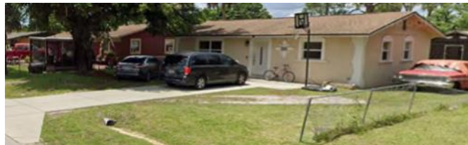
At grade home with drain under driveway
