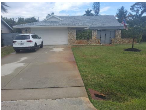
Slightly above grade home with drain in front yard
