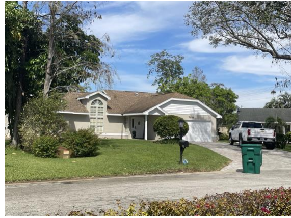
Property slightly above grade with no drainage
