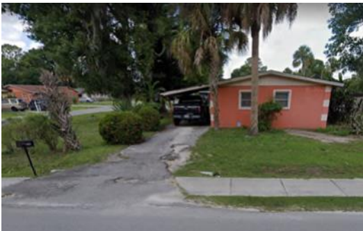
At grade home with drain under driveway
