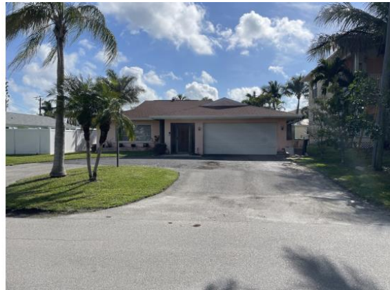
Single-family home with slab-on-grade foundation.
