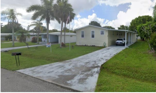
Manufactured home with drainage ditch along property and gutter that drains towards the adjacent property
