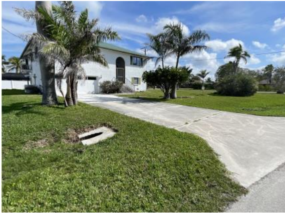
Single-family home with drainage pipe under driveway.
