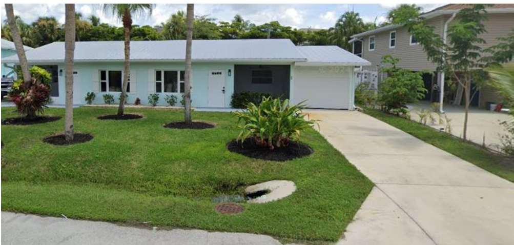
Slightly above grade home with drain and ditch in front yard
