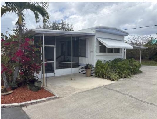
Elevated manufactured home with crawlspace
