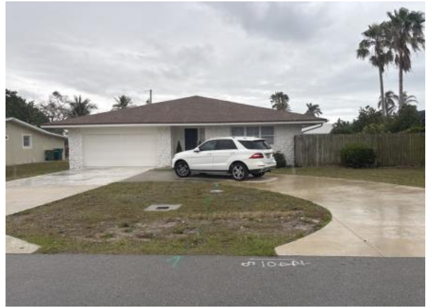
House with drainage inlet in front yard.
