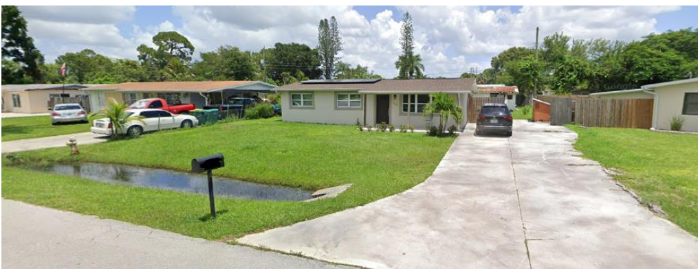
At grade home with drain and ditch
