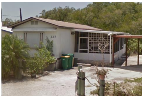
Manufactured home that has been slightly elevated.
