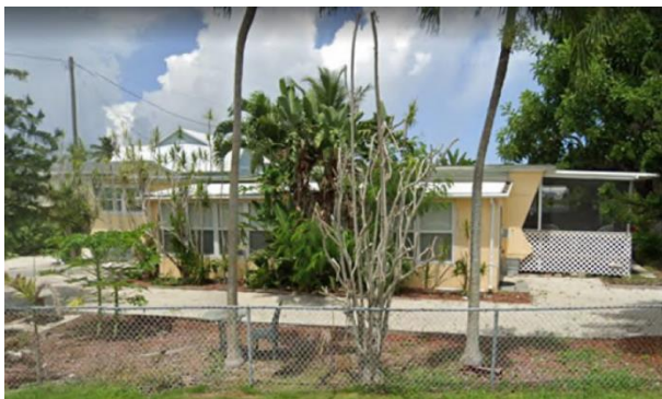
Single-family home with window-unit.
