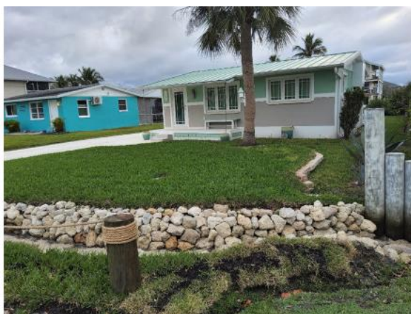
Property with drainage ditch in front yard.
