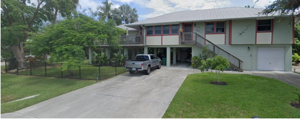
Elevated home with drain in front yard
