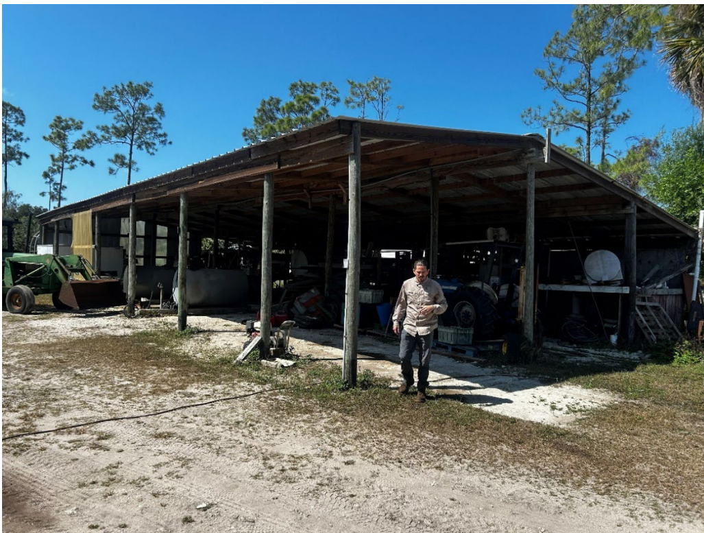
Small pole barn
