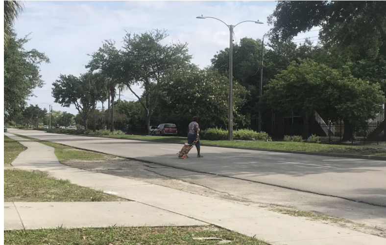
Figure 2. Double-Arm Luminaires on Concrete Pole
