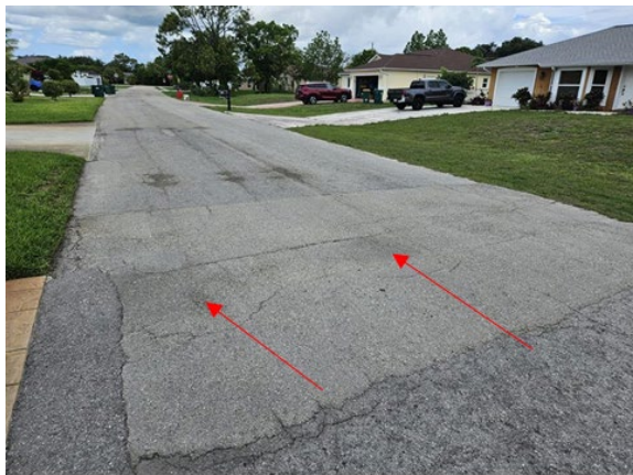
Figure 6. Bumps in Roadway
