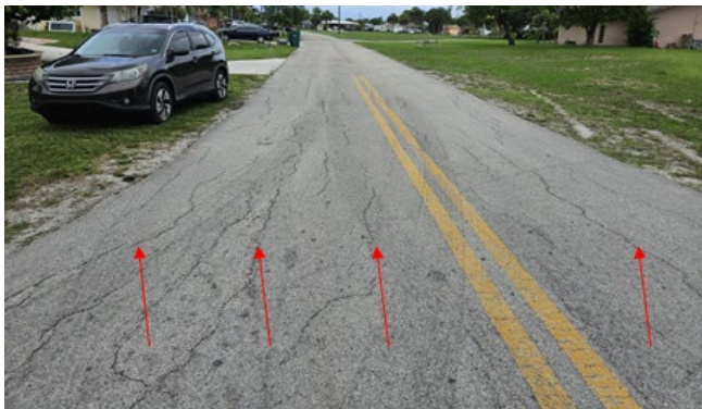
Figure 3. Longitudinal Cracking
