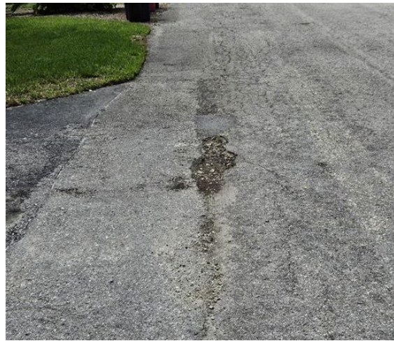
Figure 9. Pothole
