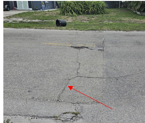
Figure 2. Transverse Cracking
