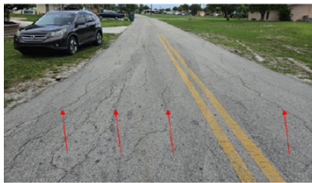
Figure 3. Longitudinal Cracking Photo location: Intersection of 17th Ct SW and 44th Terrace SW
