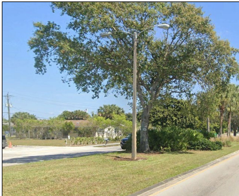
Figure 2-5: Existing Lighting East of 45 th Street SW
