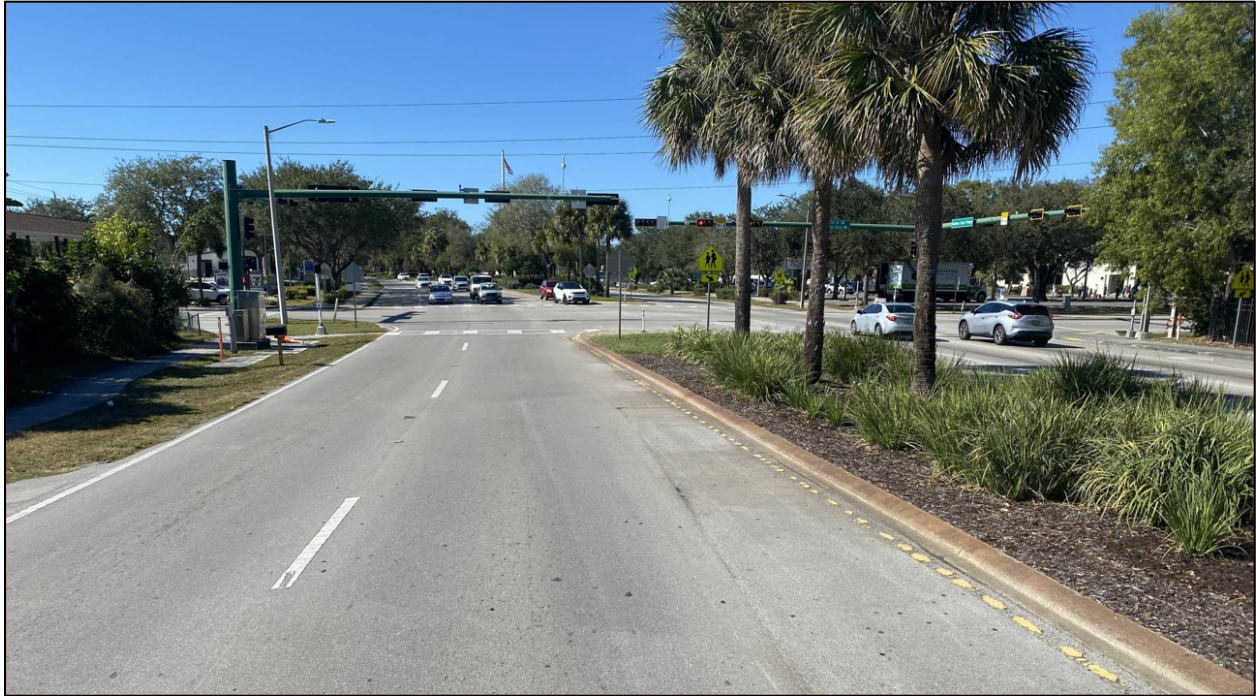
Figure 6-1: Golden Gate Parkway - Existing Roadway Conditions
