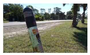
Photograph 3-5: 25th Ave. S.W. Intersection -Existing buried fiber optic cable marker
