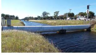
Photograph 4-4: Golden Gate Pkwy. Intersection – Looking south at existing water main crossing 951 Canal
