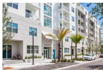
Village Place Fort Lauderdale, FL
