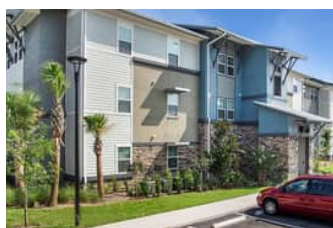
Twin Lakes II Lakeland, FL
