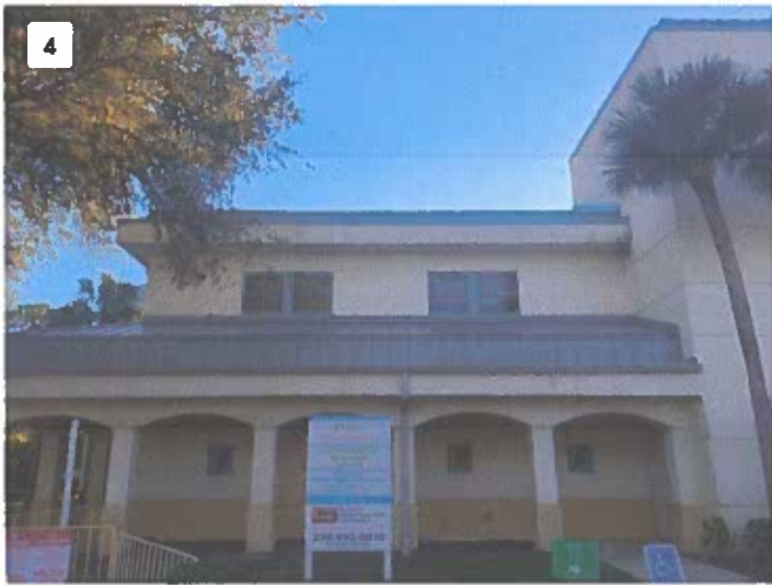
Project: Marion E Feather Window Replacement Date: Dec 30, 2025, 8:28 AM Creator: Field User
