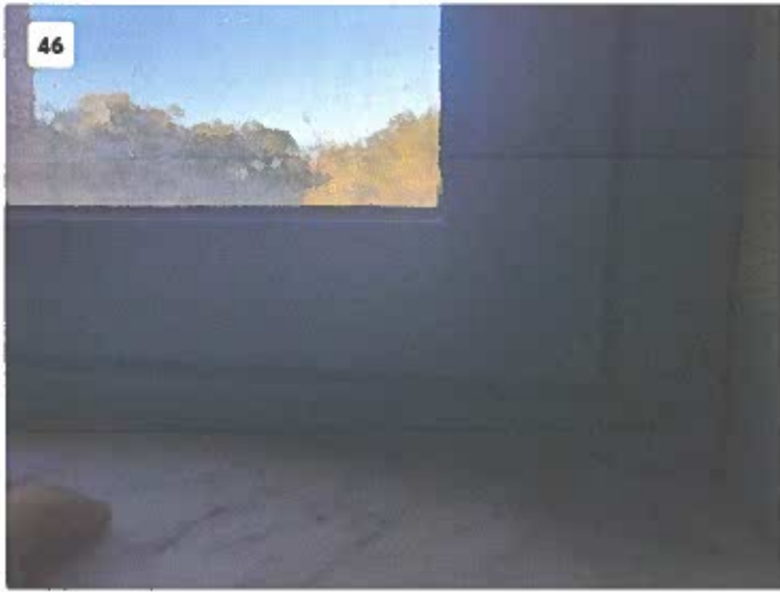
Project: Marion E Feather Window Replacement Date: Dec 30, 2025, 8:38 AM Creator: Field User
