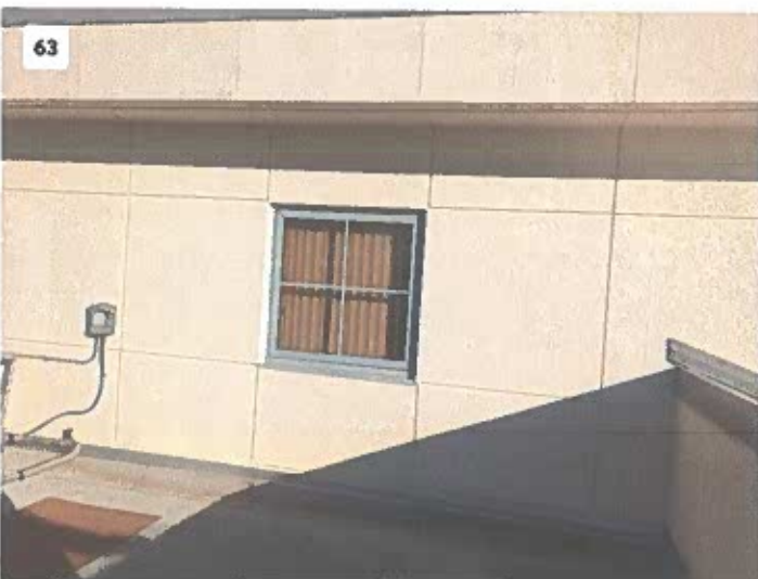
Project: Marion E Feather Window Replacement Date: Dec 30, 2025, 8:50 AM Creator: Field User
