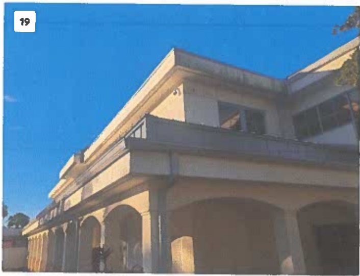
Project: Marion E Feather Window Replacement Date: Dec 30, 2025, 8:31 AM Creator: Field User
