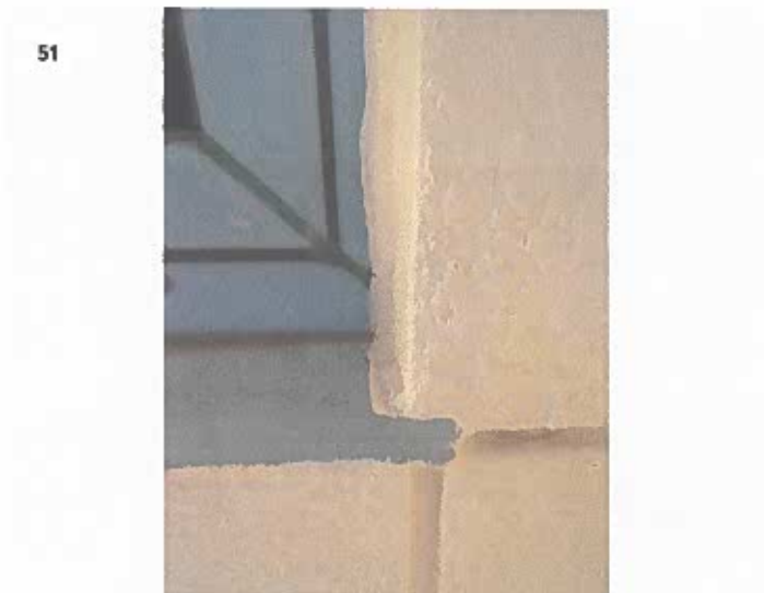
Project: Marion E Feather Window Replacement Date: Dec 30, 2025, 8:43 AM Creator: Field User
