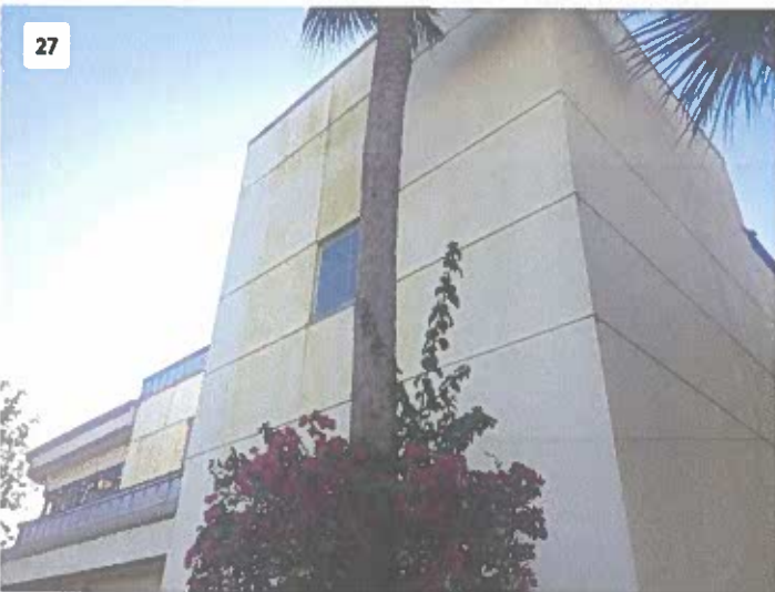
Project: Marion E Feather Window Replacement Date: Dec 30, 2025, 8:32 AM Creator: Field User
