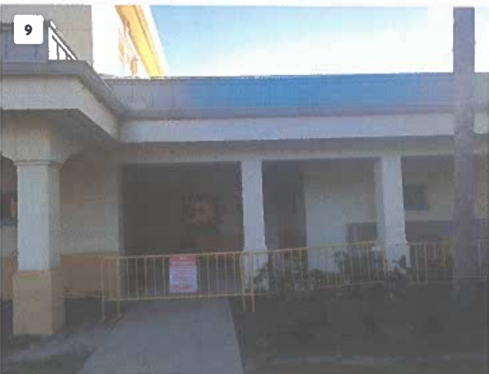
Project: Marion E Feather Window Replacement Date: Dec 30, 2025, 8:28 AM Creator: Field User
