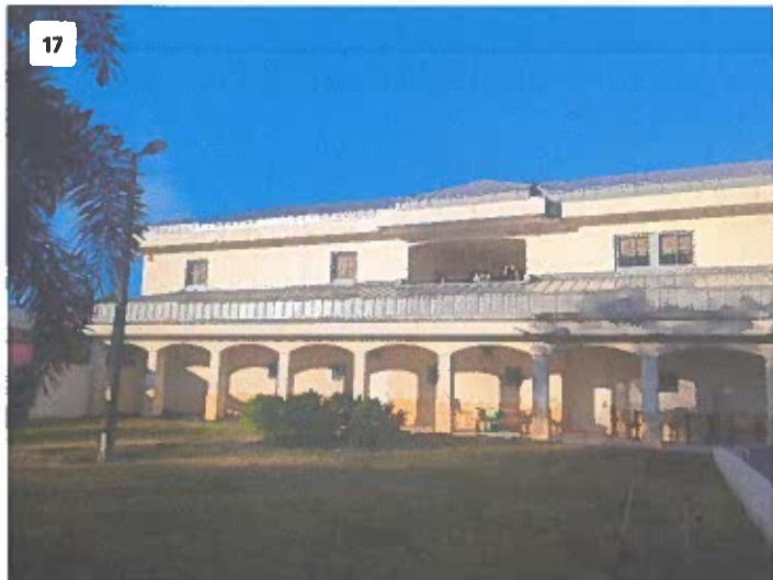
Project: Marion E Feather Window Replacement Date: Dec 30, 2025, 8:31 AM Creator: Field User
