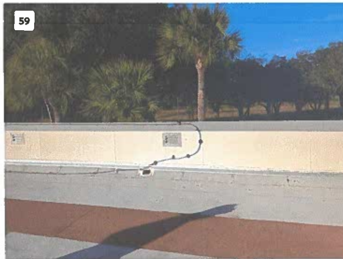
Project: Marion E Feather Window Replacement Date: Dec 30, 2025, 8:47 AM Creator: Field User
