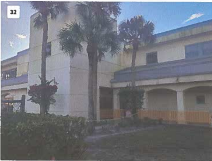
Project: Marion E Feather Window Replacement Date: Dec 30, 2025, 8:33 AM Creator: Field User
