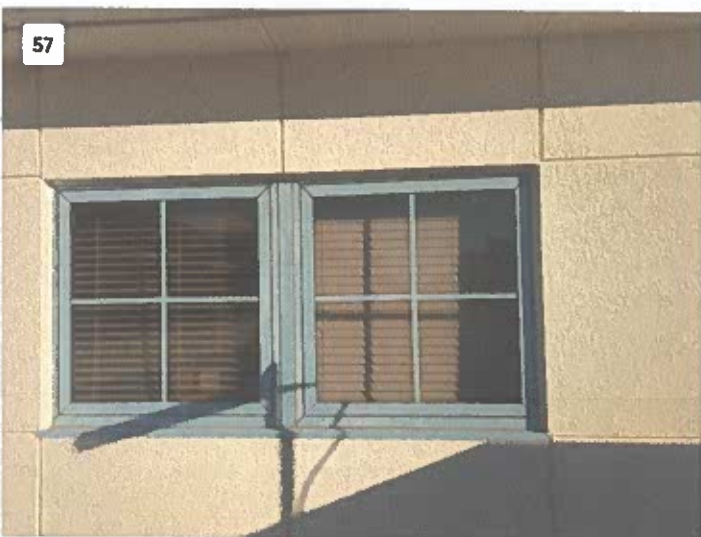
Project: Marion E Feather Window Replacement Date: Dec 30, 2025, 8:47 AM Creator: Field User
