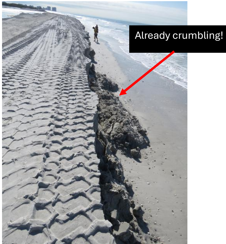
New Berm, where there was previously a Loggerhead turtle nesting beach.
